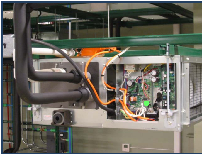
Fan Coil Control PCB
