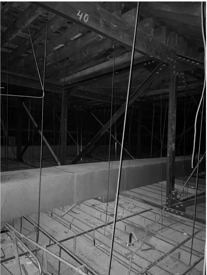
PHOTO - EXISTING PLASTER CEILING PLENUM
